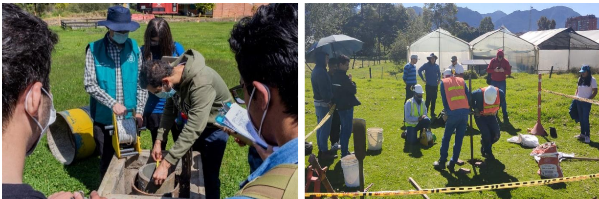
Figure 3. Activities developed in the Bogota Campus. A) Students measuring the casing diameter of a well before take groundwater levels B) Monitoring well construction with the presence of geology and engineering students.
